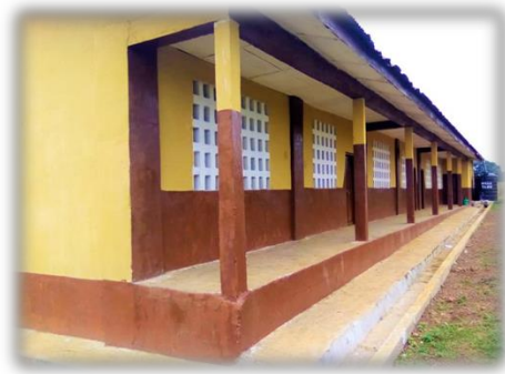
Koinadugu II Primary School (post-intervention)
