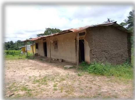
Mbaoma Lutheran Primary School (pre-intervention)
