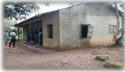
Foya RC Primary School (pre-intervention)
