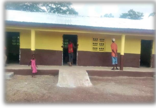
Kantimpie WCSL Primary School (post-intervention)
