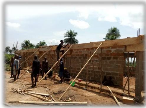
Kantimpie WCSL Primary School (during-intervention)
