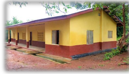
Foya RC Primary School (post-intervention)
